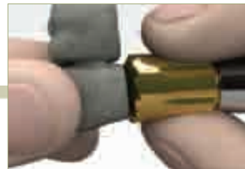
Eliminate the Lip remnant caused by 'snap-on' mechanism by reamer
